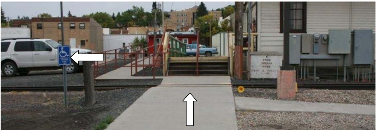
Above Photo Description: Handicap parking and access to AMTRAK station. Passengers must cross BNSF's house track for station access.
